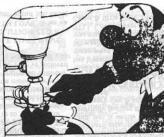
4) The foreign matter has accumulated in the elbow joint, or trap; I take apart the joint.
